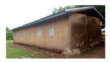
On the side, where the plaster has crumbled away, you can see the wall made of pounded clay.
