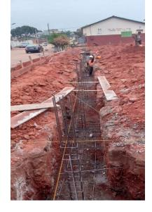
The second reinforced concrete layer is poured on top. Once it has dried, the foundation walls are built on top.
