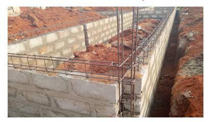
The walls of the building are built on top of the iron anchor. When the walls reach the height of the window openings, a small iron anchor is inserted.
