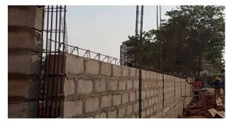
The walls then quickly rise to the window lintel. After the pillars on the veranda are cast, the upper iron anchor is placed, sheathed, and cast in one piece.
