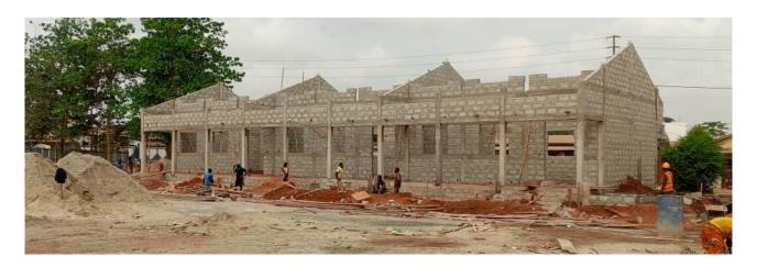
The walls now need to dry for about three weeks before the roof can be made. We estimate two weeks for the roof to be completed. Immediately afterward, the plastering and cementing work will begin, which we estimate will take between three to four weeks. The plaster will then dry for another three weeks before the paint can be applied.
