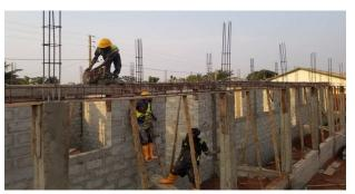
The walls are then raised by 4 rows of bricks before the fourth iron anchor is cast below the roof.
