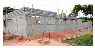
A fourth iron anchor is cast below the roof before the gables are erected on it. Finally, the ends of the pillars are boarded and cast.
