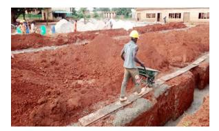
The iron base for the foundation is placed on the first reinforced concrete layer and the iron inlays of the pillars are incorporated into it. They are all lined up neatly with the help of cords.
