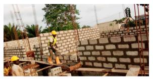
A small iron anchor is incorporated below the window openings and then the walls are erected up to the window lintel.
