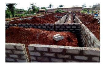
The iron inlay for the lower iron anchor is placed. Then the lower iron anchor is cast. The walls of the building grow on top.
