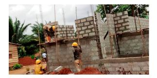
The pillars of the building and the veranda are being poured. In order to save boarding wood, we had metal molds made for the pillars of the veranda.
