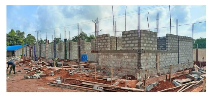
While the carpenter prepares the formwork for the upper iron anchor, the bricklayers build the ramp and the staircases.
