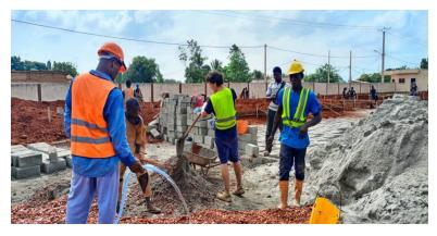
The second layer of concrete is poured over the iron reinforcements. The foundation walls are then built on top. The lower iron anchor is poured, and the building's walls are constructed on top of this.
