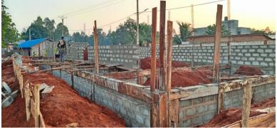
When the walls reach the height of the window openings, a small iron anchor is cast there.
