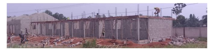
The walls are now raised by four rows of bricks before one more iron anchor is made below the roof.
