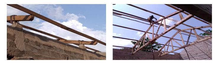
The entire roof structure is finally attached to the building with smooth iron rods.
