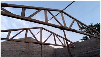
The cross ties are lashed by means of the iron rods of the pillars. The longitudinal planks are attached.
