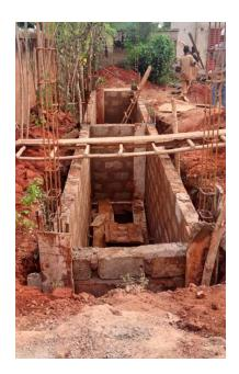
The toilet pit is plastered using sikalite and sikalatex and then closed.
