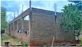
The window openings are too wide and there is no iron anchor below the window openings, the doors are too low, the building structure is good.
