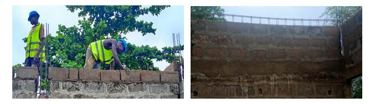
After the iron anchor has been cast, the gables are built.
