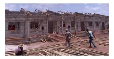
The longitudinal beams are attached above them and the asbestosfree Eternit panels are screwed on.
