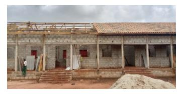
Once the roof is finished, the plastering work begins, first inside the rooms and then outside.
