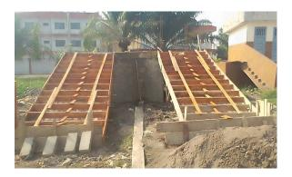
A large top slab is poured to provide space for the stairways.
