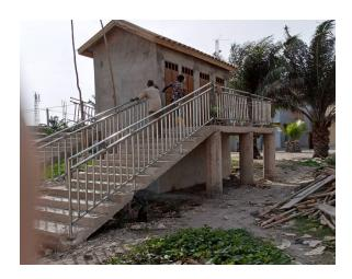
The toilet house is built above this. Since the school is not far from the sea, we put on a roof made of Eternit panels. Corrugated iron would rust too quickly in the salty air. The railings are installed.
