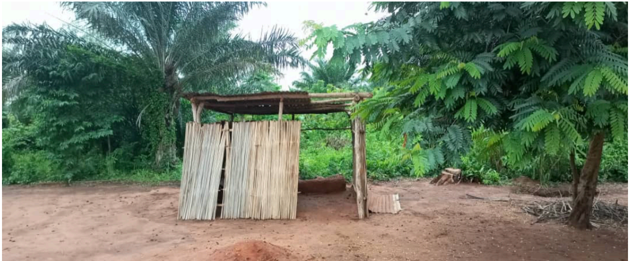
The kitchen of the canteen.
