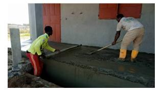
With the water removed from the toilet pits, the masons were able to level the ground and pour the reinforced concrete slab and build the walls on top.
