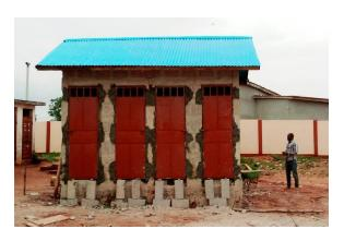
After the walls of the building had dried well, the carpenters made the wooden roof structure and put on asbestos-free panels.
