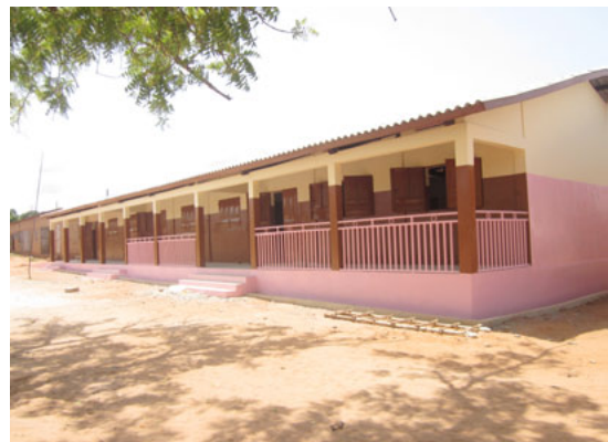
The building of the Public Primary school of Dekanme is ready for the children to move in.
