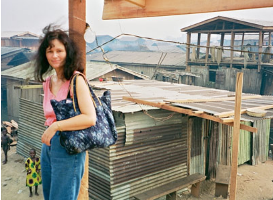
Astrid single-handedly on the construction site of the Primary School of Makoko Waterside in Lagos, Nigeria, a school for Beninese economic refugees.
