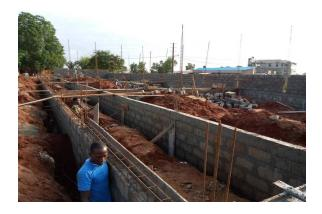
The lower iron anchor was poured and the walls of the building were built on it. The walls quickly grew up to the window openings. At the same time, the pillars were cast on the veranda. In order to use less wood, we had molds made of metal.
