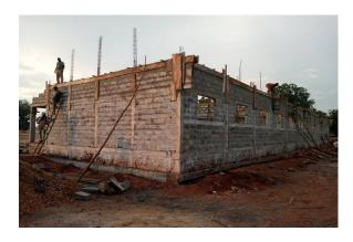
After the upper iron anchor, another additional ring anchor was cast below the gables, so that the building would gain a bit in height. Then the gables were erected and the shutters inserted.
