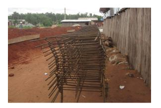
The foundation underlayer was poured into which the iron inlays of the pillars were incorporated. The foundation walls were built on this.
