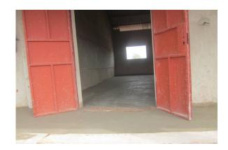
As soon as the roof was made, the plastering work was started and the floors were cemented.
