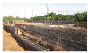
The buildings are situated on a slope. Therefore the foundation had to be anchored once in between. Only after that the usual lower iron anchor could be cast. The walls grew on it and the small iron anchor below the window openings was cast.
