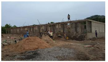
The gables were erected on the iron anchors, the stairs were made.
